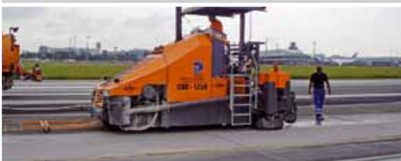
Grooving, Grinding, Scoring mit BumpCutter Grooving, Grinding, Scoring with BumpCutter
