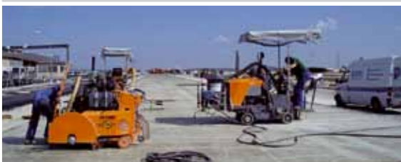
Fugenschneiden Joint sawing
