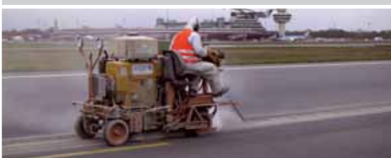
Demarkieren Removal of airport markings
