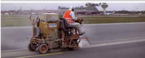
Demarkieren Removal of airport markings
