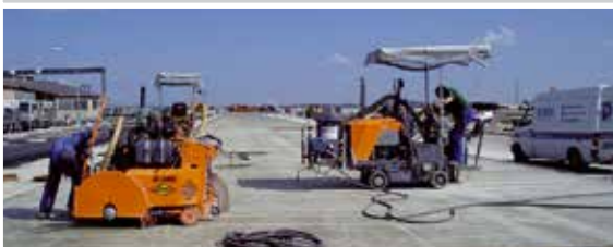
Fugenschneiden Joint sawing
